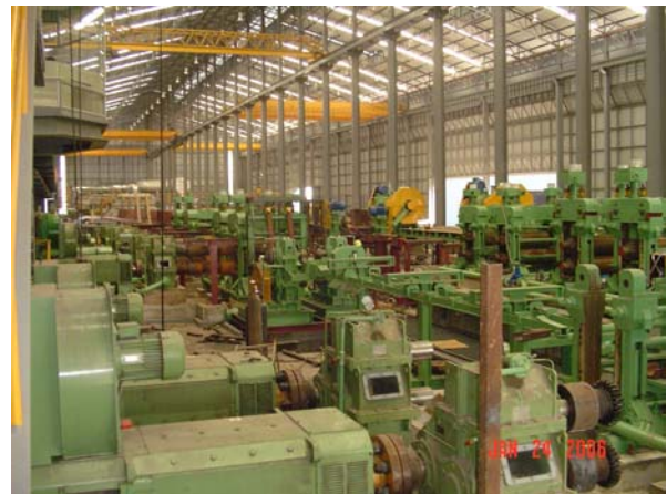
Figure 8-RM2 Intermediate Stands during construction
