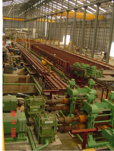
Figure 7-RM2 Shears and Cooling Bed during construction
